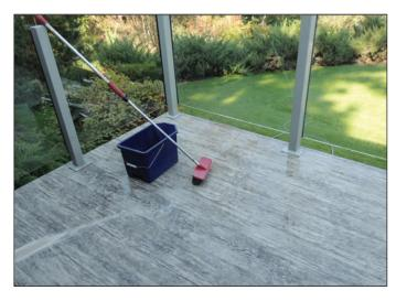
Pressure washing equipment can severely damage vinyl deck membranes if not used with caution. If a pressure washer is used please keep the following items in mind:
