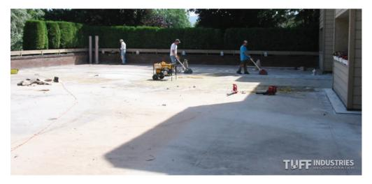
Tuff Industries recommends that all installation surfaces are completely free from synthetic compounds such as chemicals, sealants, or coatings. Avoiding substances that could affect the bond of the Tuff branded vinyl deck membrane is critical to the product's long term performance. Existing coatings or contaminates could also cause discoloration or premature aging of the Tuff vinyl decking product.
