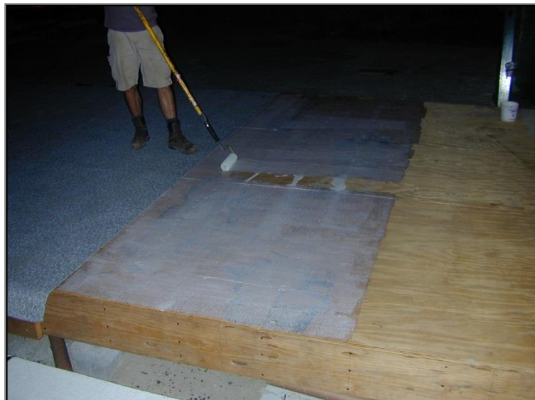
View of Adhesive / Membrane Application
